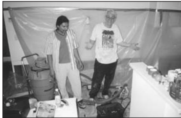
Lance helps workman from Jordan Environmental, Inc. to repair damage.
